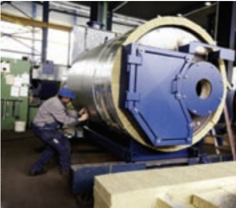
Insulation works on a fire tube boiler with Rockwool Duraflex
