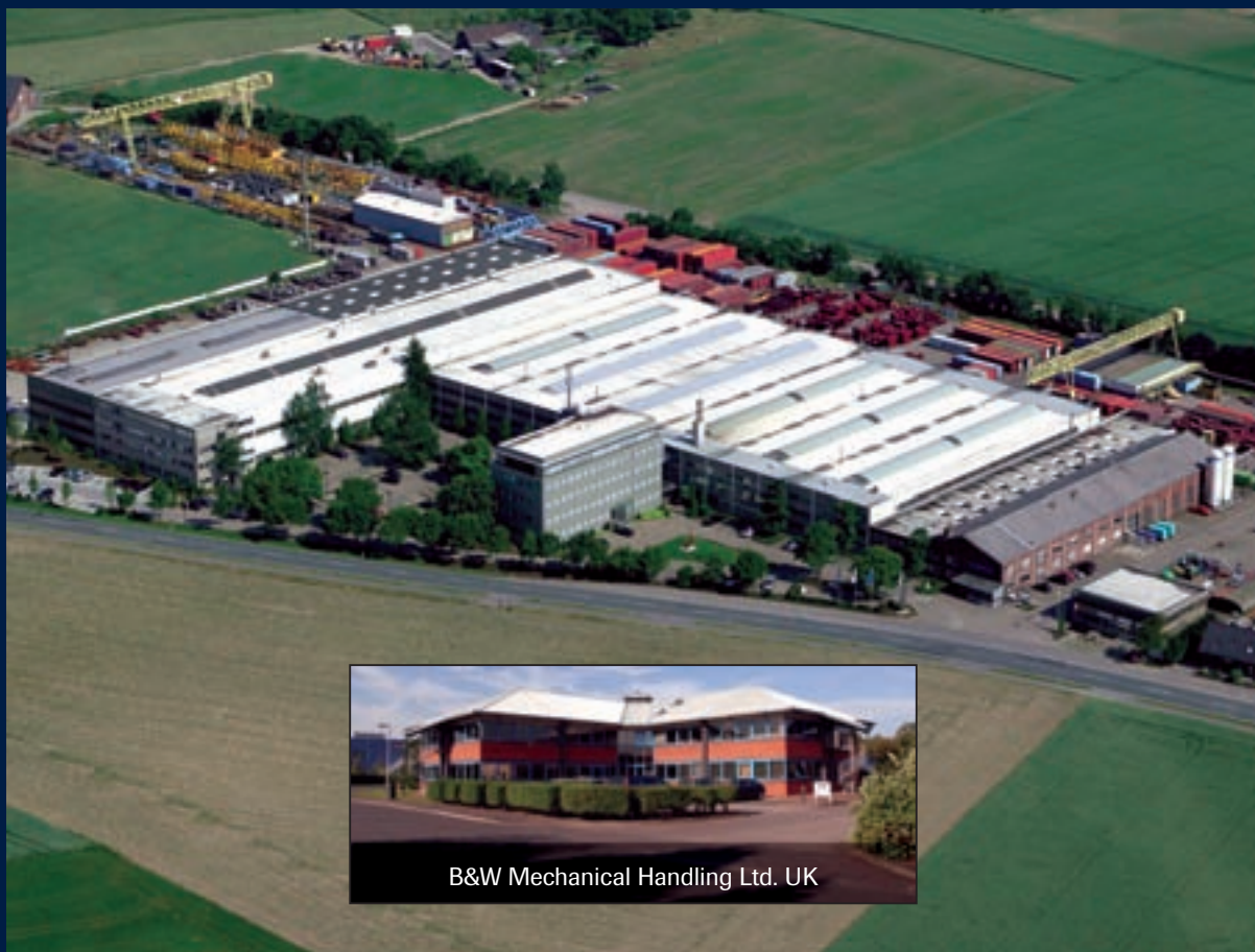
AUMUND GROUP Headquarters in Rheinberg, Germany
