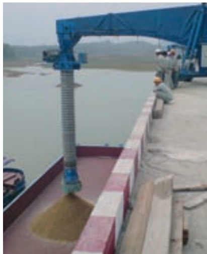
Shiploader with Enclosed Boom and Telescopic Free Fall Chute
