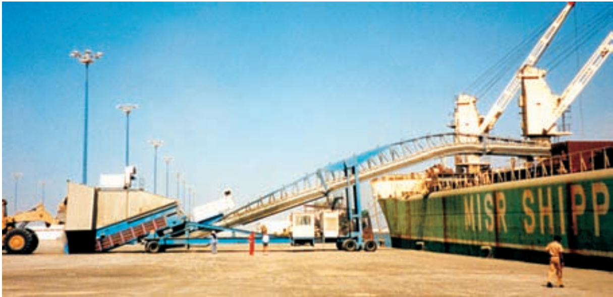
Full Specification Shiploader handling Cement Clinker to Handy Size Ships
