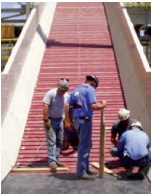
Illustrated above the B&W site supervisor demonstrates the proper fitting of the conveyor belt over the Samson™ Apron-Bars.
