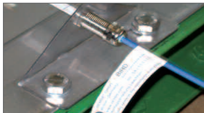
BIRD (Burst Indicator REMBE® design) – retrofittable
