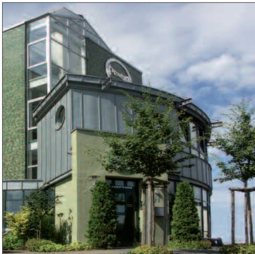
REMBE®-headquarters in Brilon / Germany
