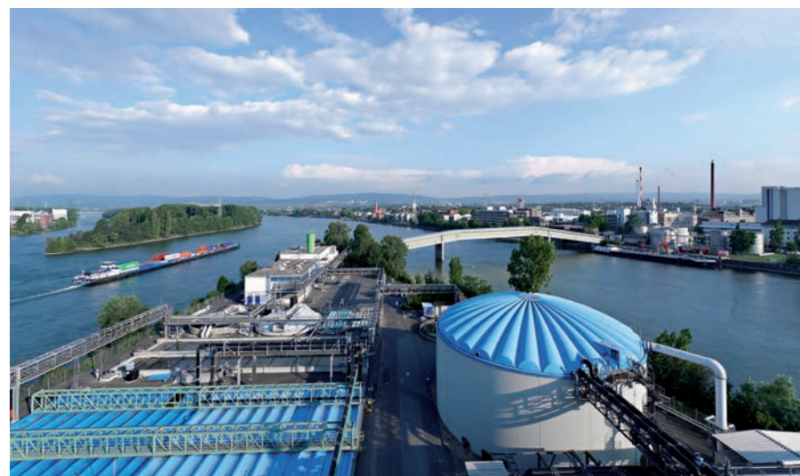
As part of the strategic development cooperation between SAMSON and InfraServ Wiesbaden, the two companies launched a joint pilot project to optimize the processes in the biological water treatment plant in the industrial park. ©InfraServ Wiesbaden
