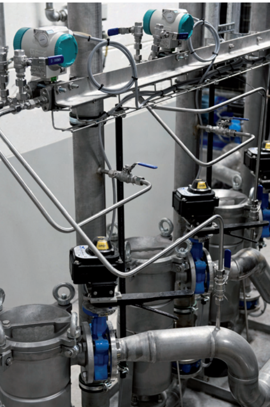
The pressure transmitter P DS III in the mode differential pressure measurement.
