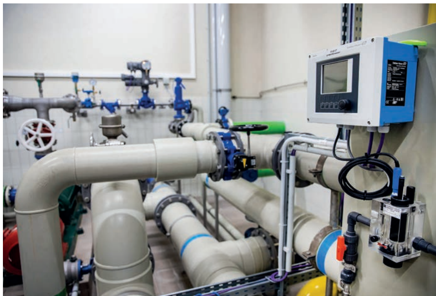
The pH value is also measured as part of the quality analysis during treatment of the raw water for the potable supply network.
