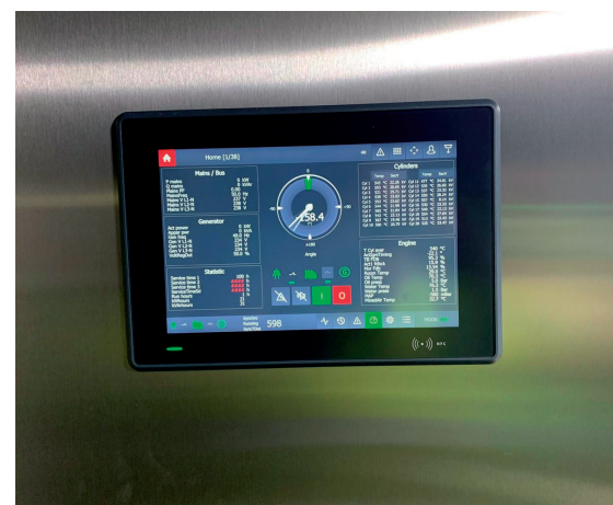
The vandalised control screen and the Motortech replacement with touchscreen.
