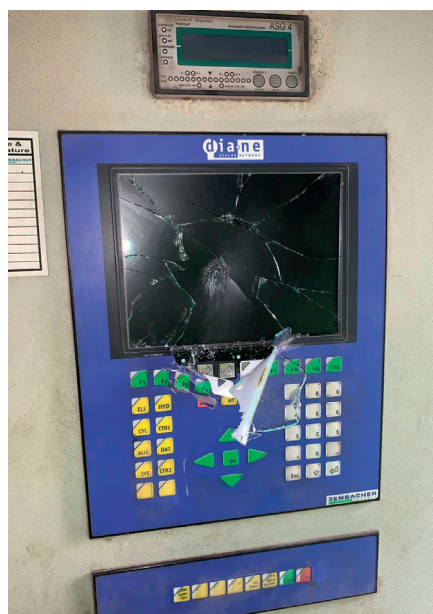
The vandalised control screen and the Motortech replacement with touchscreen.
