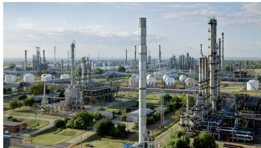
Implementing standardized asset integrity procedures can not only drive production efficiency, but improve safety and reduce risk as well.
