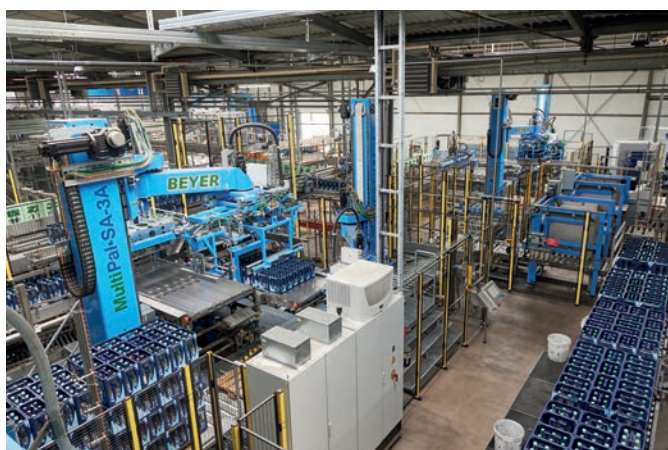
View of the palletizer technology in the new glass system.
