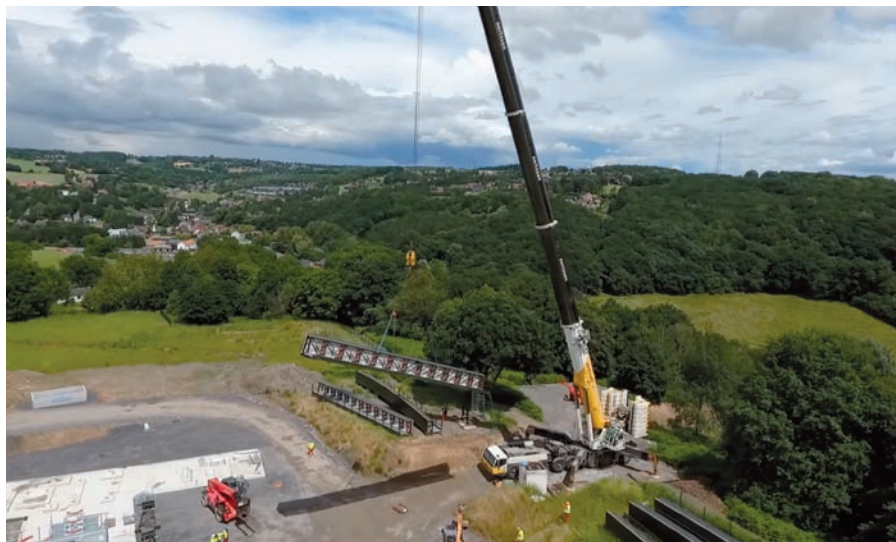
Demanding assembly work to get the conveyor operational
