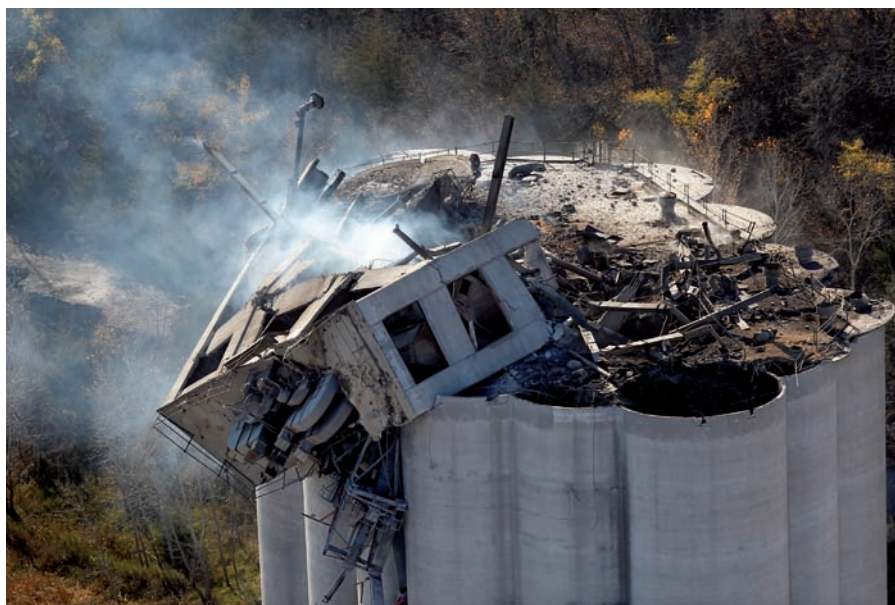
2011 Barlett Dust Explosion - originated in Bucket Elevator
